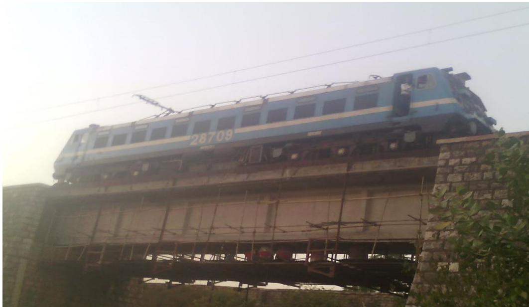
Figure 4. Actual load has applied to the for monitoring before strengthening
