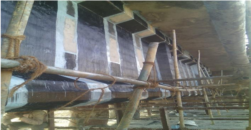
Figure 8. U-wrap FRP applied to PSC I girder
