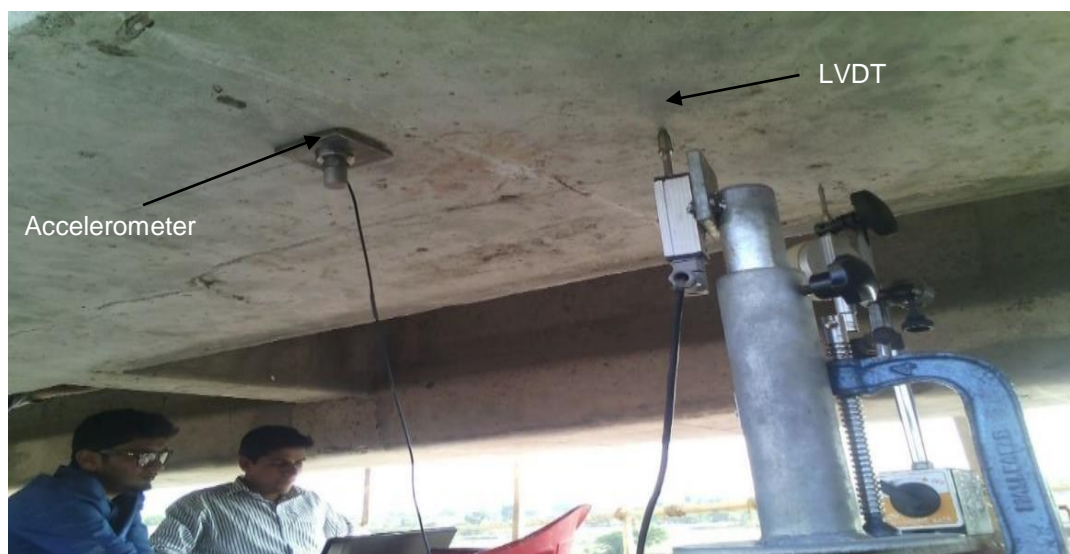
Figure 3. Structural health monitoring of Ratlam railway bridge with help of sensor
